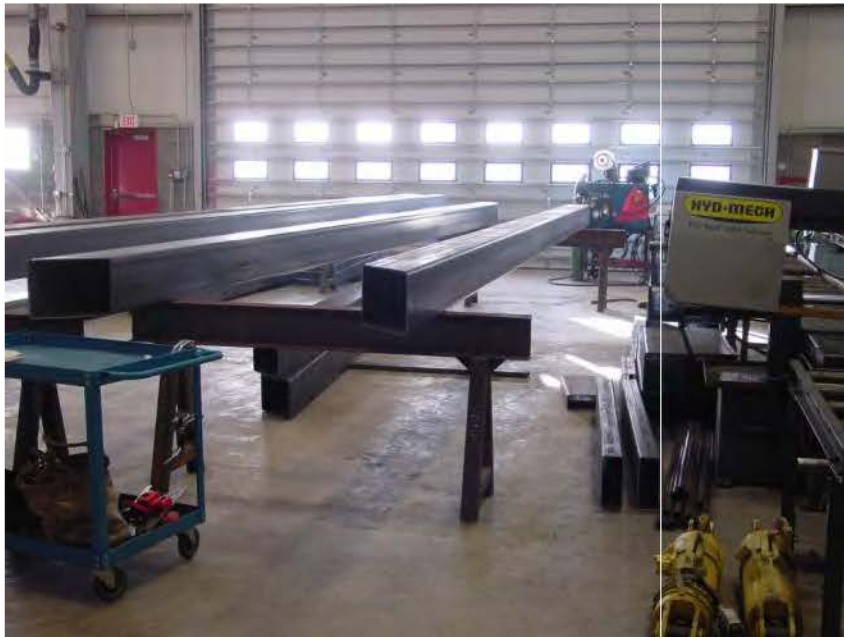
Construction of DWRC at the Mammoet facilities in Canada
