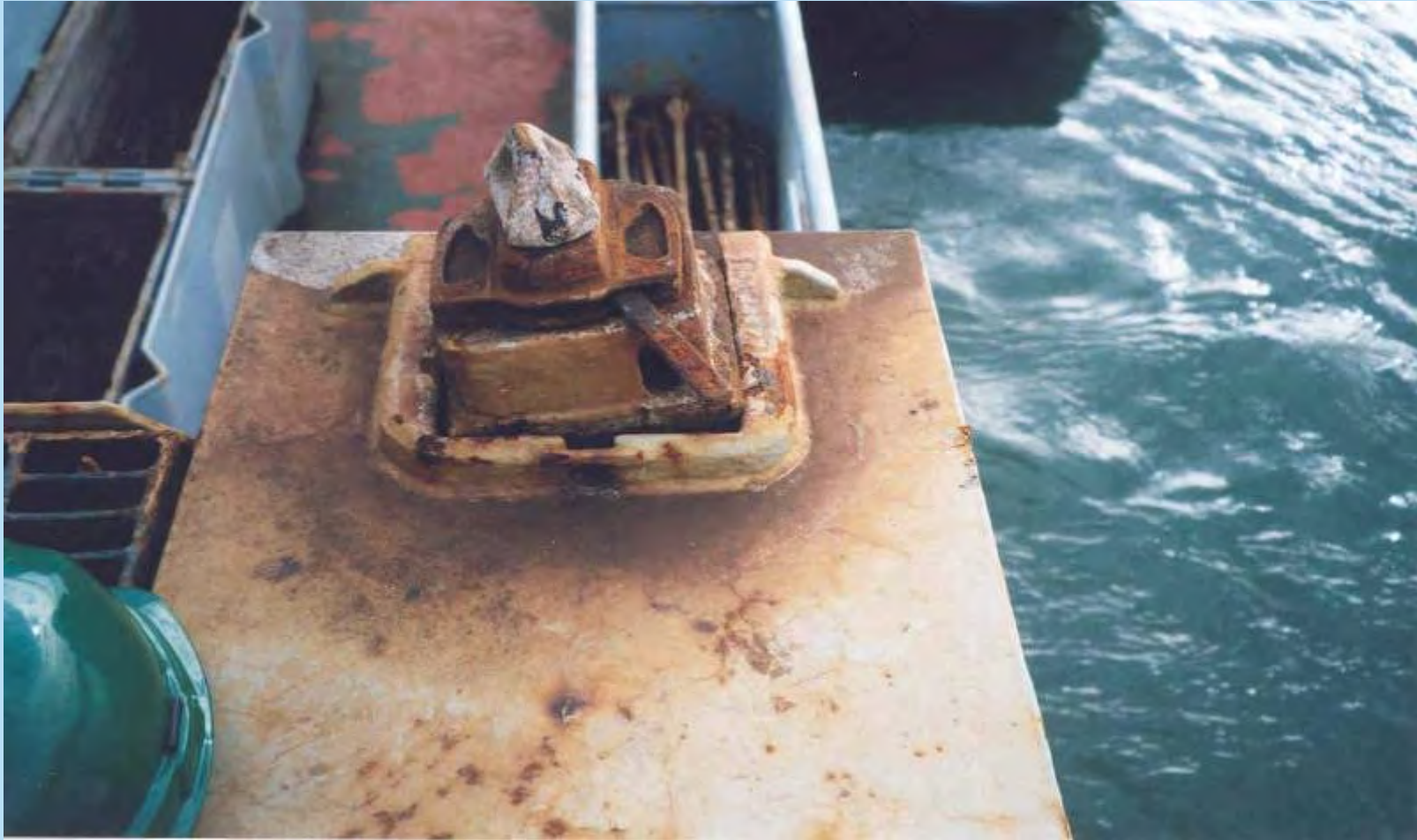
Poor condition of twistlocks, bottom foundations
