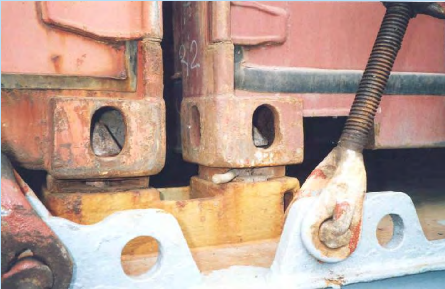
Poor condition of twistlocks, bottom foundations
